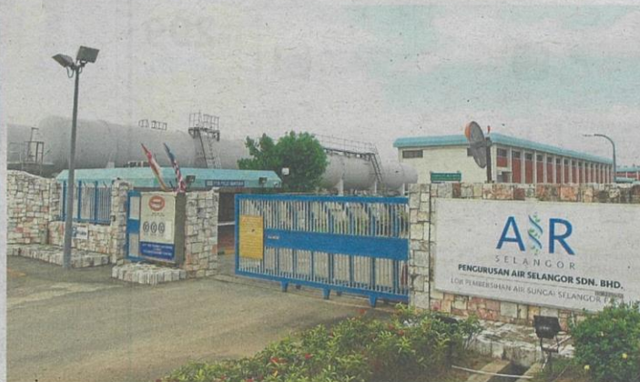
Upgrading works at the Sungai Selangor Phase Two Water Treatment Plant led to the scheduled water cut last month. — Filepic
